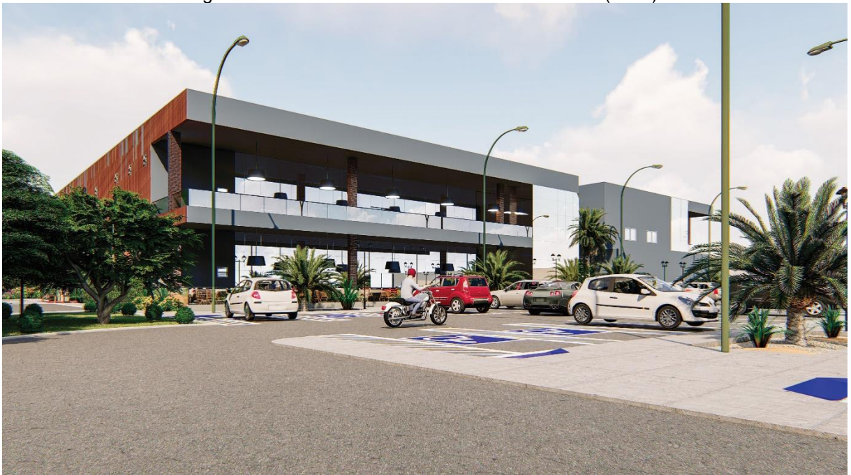
Figura 52: Fachada Lateral Restaurante Maracani (2020).
