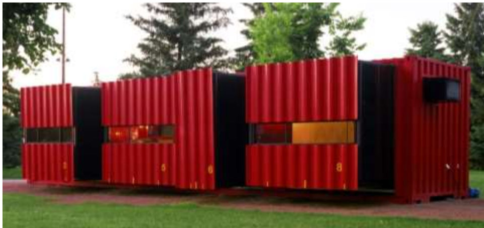
Figura 03: Vista Externa do Mobile Dwelling Unit
